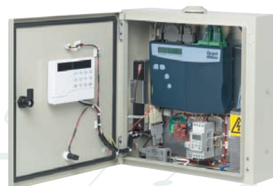
Squirrel 2020 in an electrical enclosure
